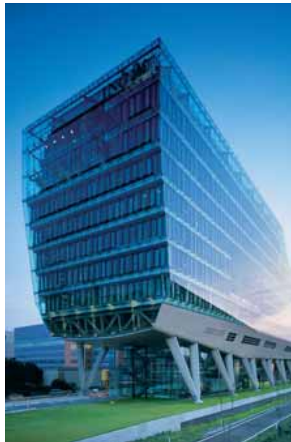
ING House, Amsterdam, Niederlande ING House, Amsterdam, The Netherlands
