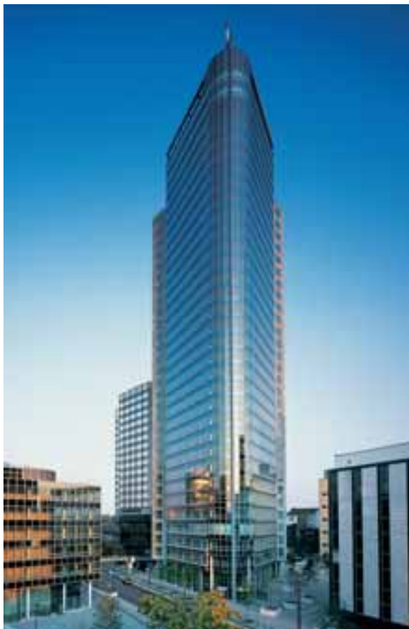
CityTower, Offenbach, Deutschland CityTower, Offenbach, Germany
